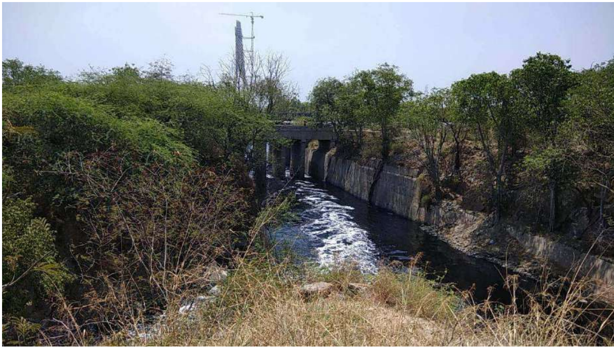
Fig. 2.8 Nazafgarh drain joining Yamuna River near Signature Bridge, Delhi
