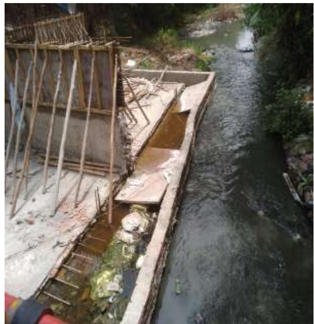
Weir is being constructed
